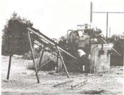
Obsolete jaw-crushers in the copper leaching plant. These low-capacity crushers reduced the ore to minus \frac{3}{4} in. for heap leaching.
